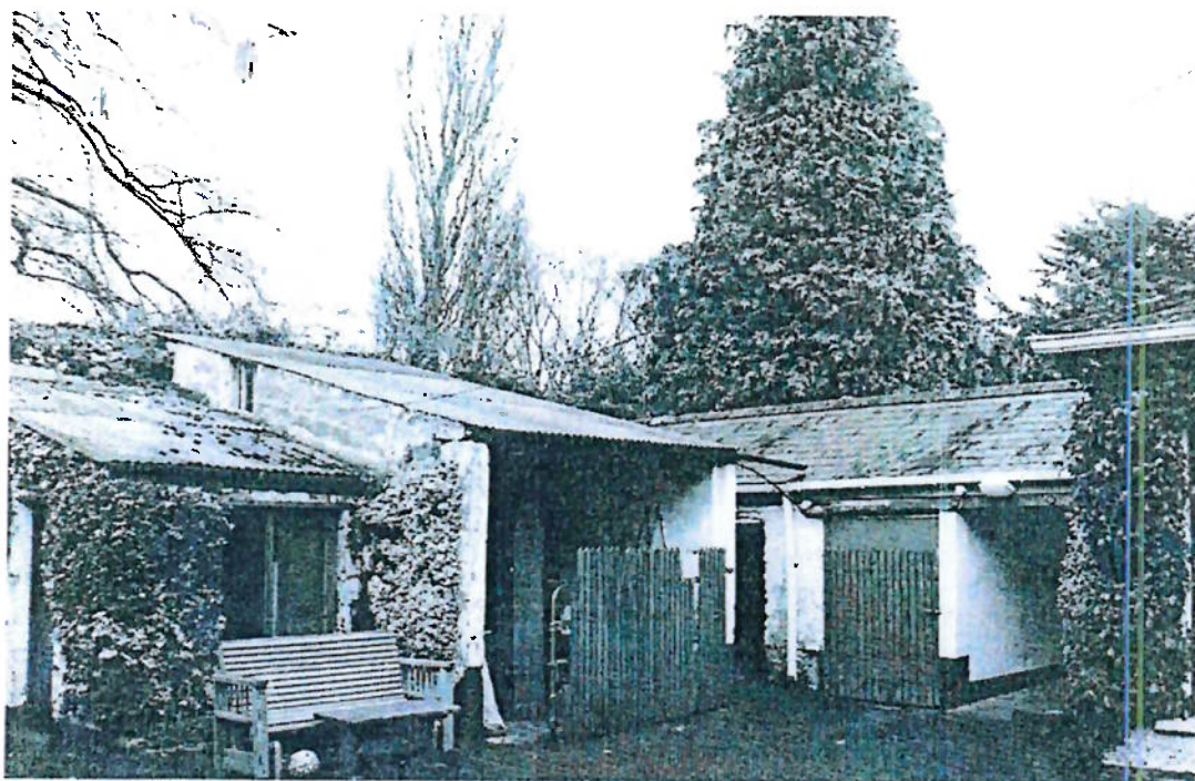
fig 20 Outbuildings to north of house
