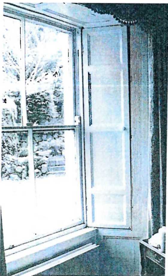
fig 15 Shutters in south bow showing fluted detail.
