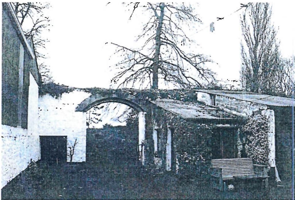
fig 18 Entrance arch to rear yard.
