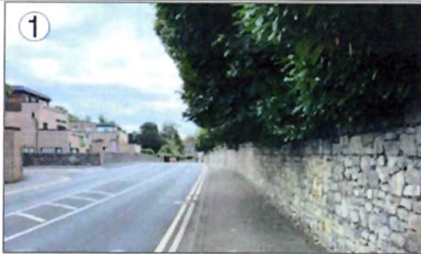
Figure 5: Photo 1 view of wall -current curtilage wall for Portrane House (Source: Design Statement by van Dijk Architects)
